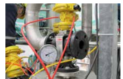
Slaughter house piping cleaning
