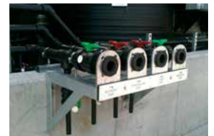
Chemical discharge area
