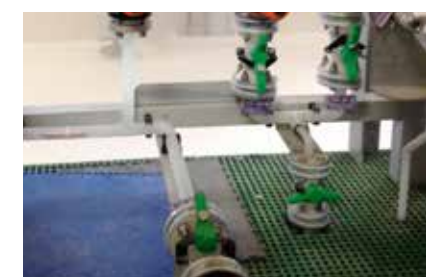
Anti-scaling unit (H 2 SO 4 96%)
